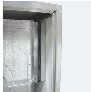
Sealing on the outlet side.
